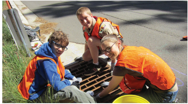
Boy Scouts help mark storm drains in the Sierra Tract neighborhood with AmeriCorps Member Brenna Blessing.
